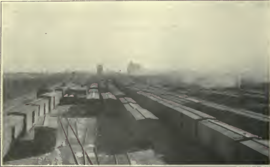
FIG. 331. FREIGHT YARDS. Galewood Yard of the Chicago, Milwaukee & St. Paul Railway.
